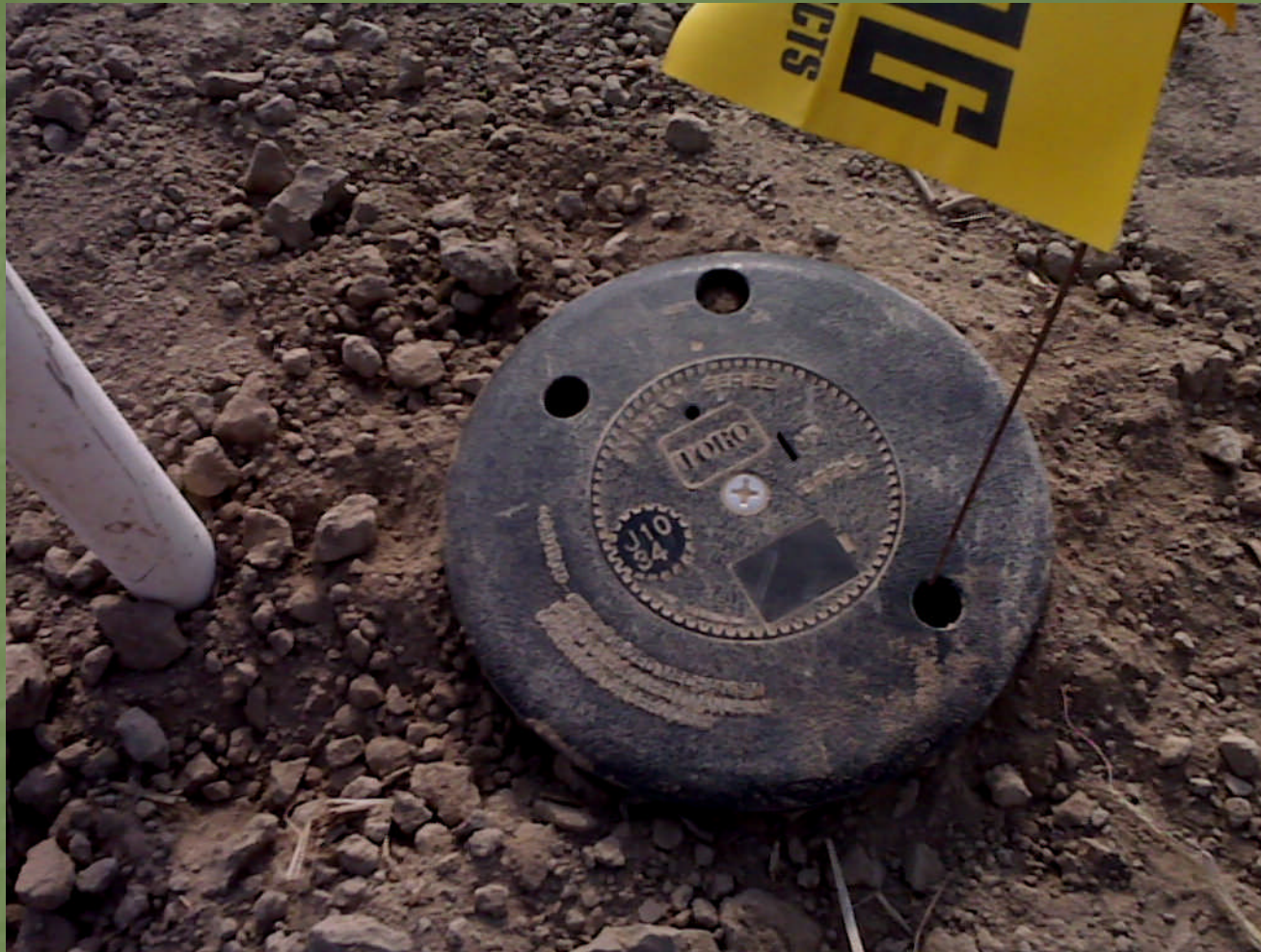
Irrigation Head Installed
