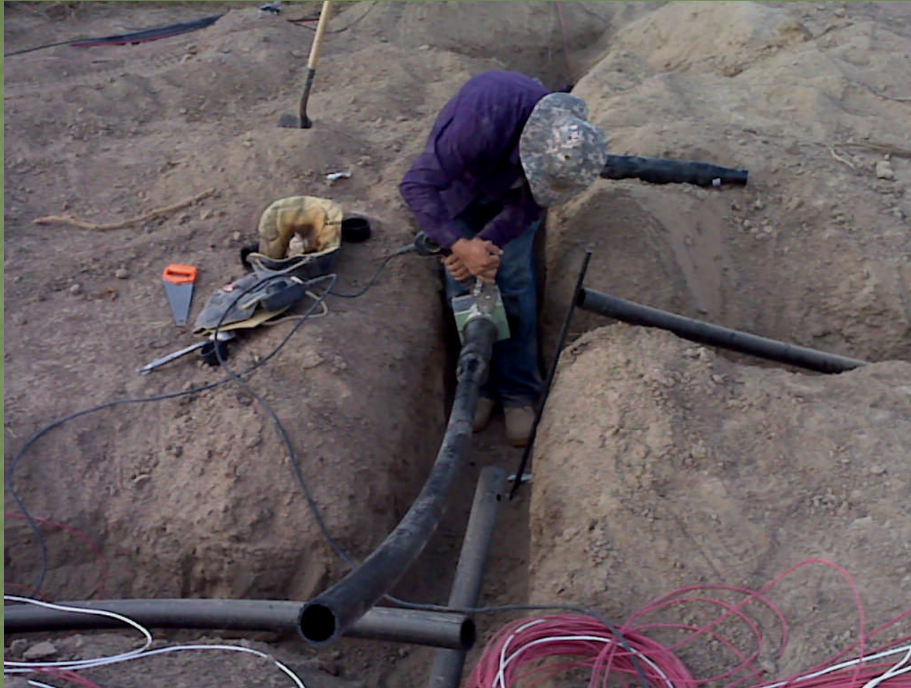
Fusing HDPE Irrigation Pipe
