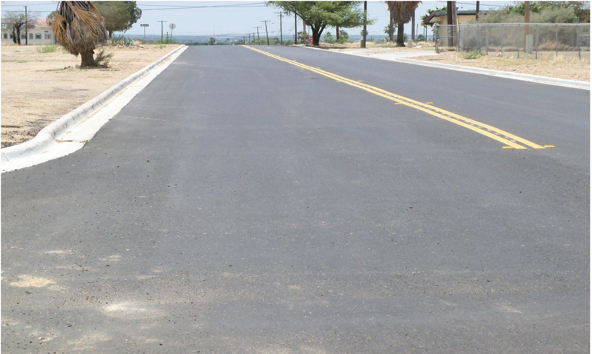
Pappas Street **West view from Thomas Avenue
