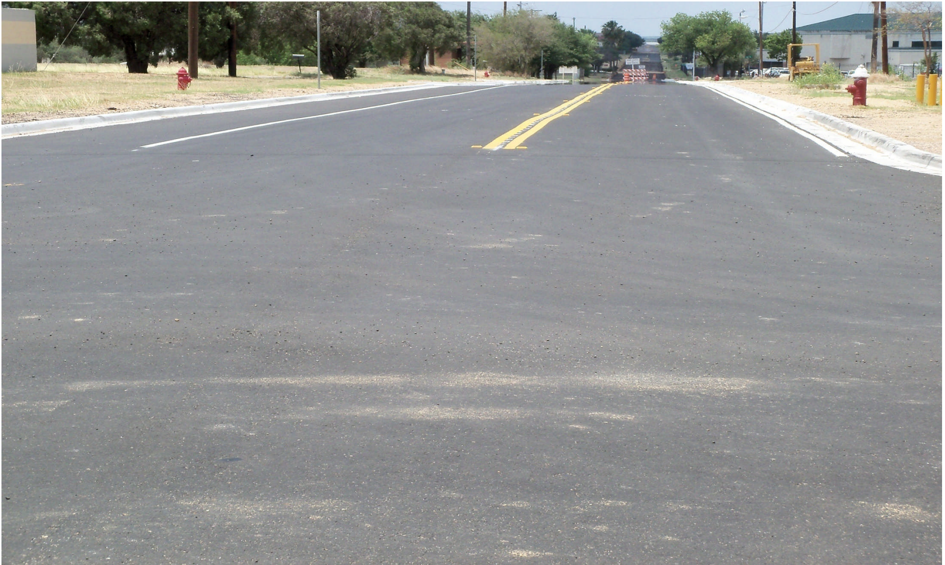
Thomas Avenue Industrial Street Reconstruction. **Looking north from Pappas Street intersection.
