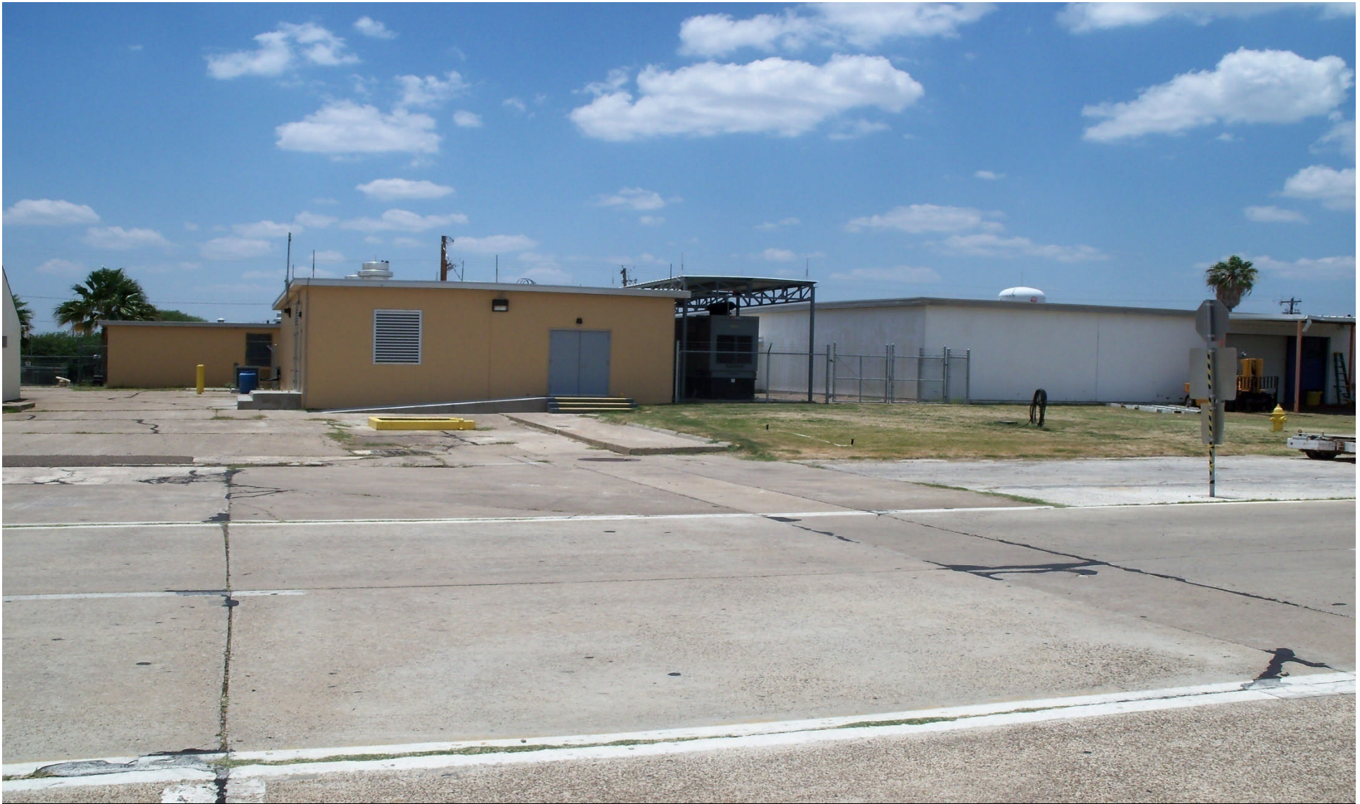
Rehabilitated Airfield Electrical Vault
