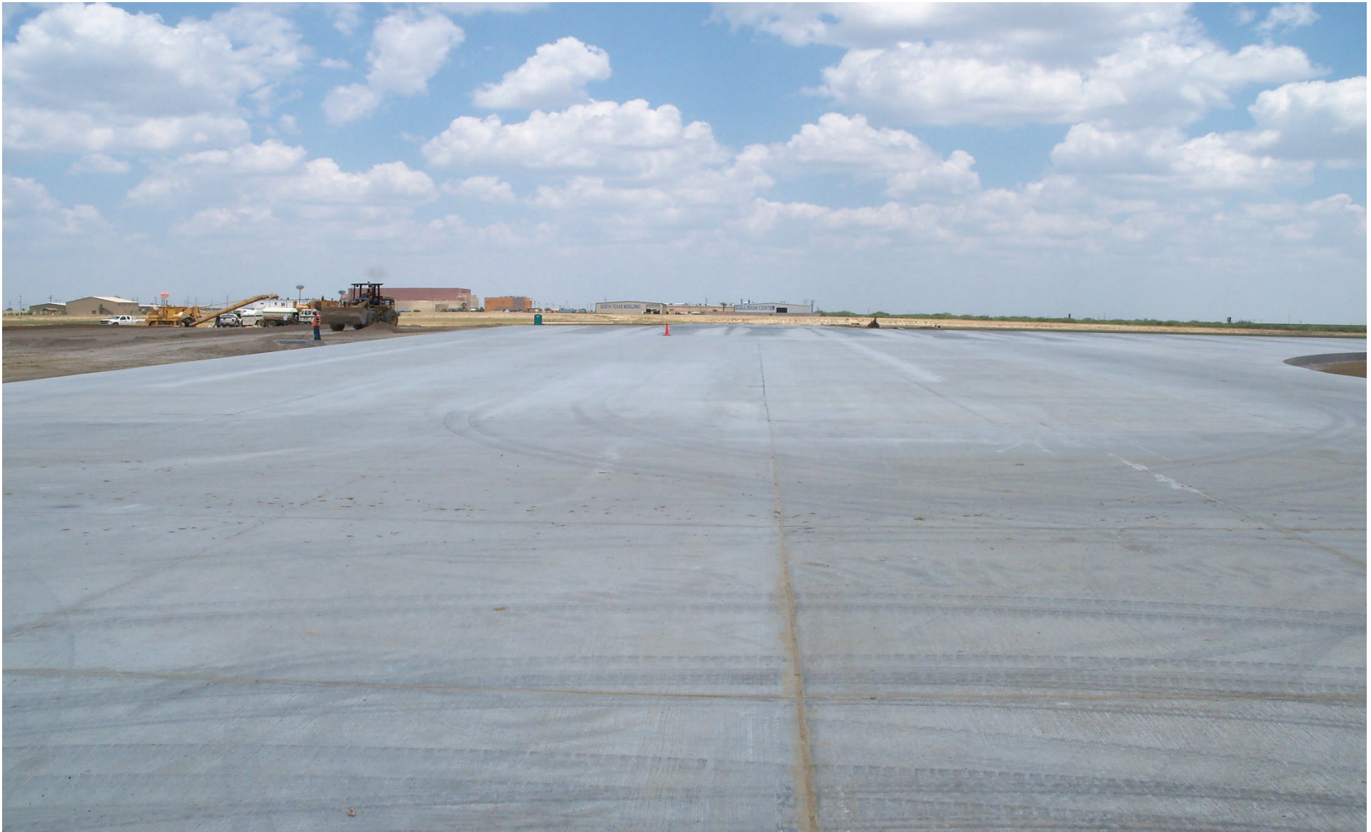
Reconstructed Taxiway "A"
