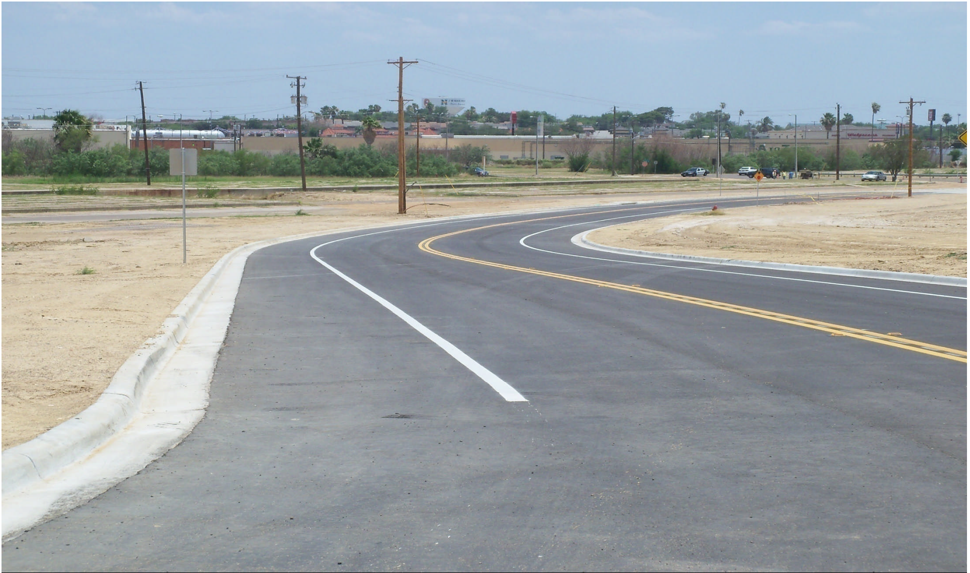
Thomas Avenue Extension ** View from Pappas intersection looking south to Bustamante Ave.
