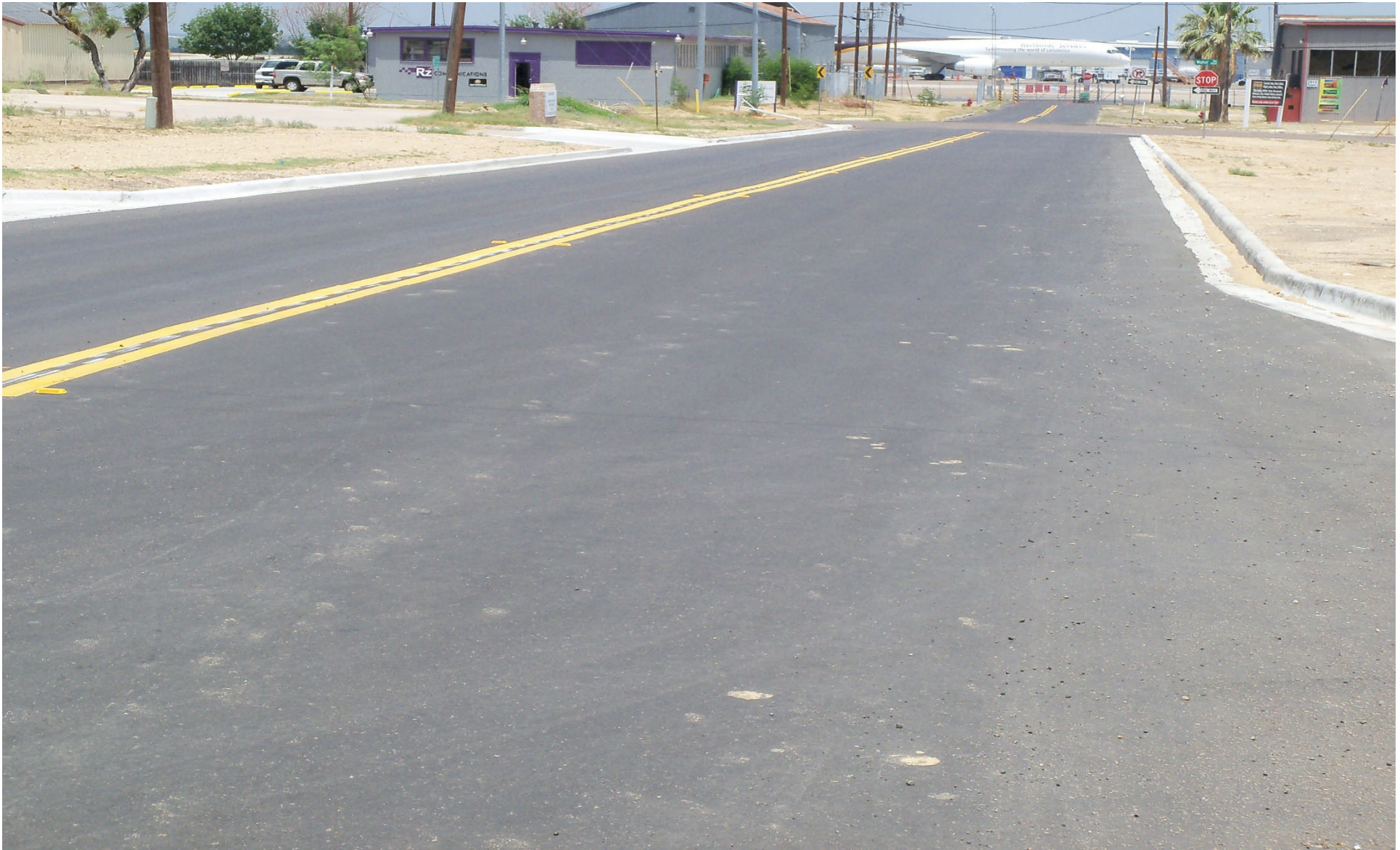
Pappas Street Reconstruction **East view from Thomas Avenue
